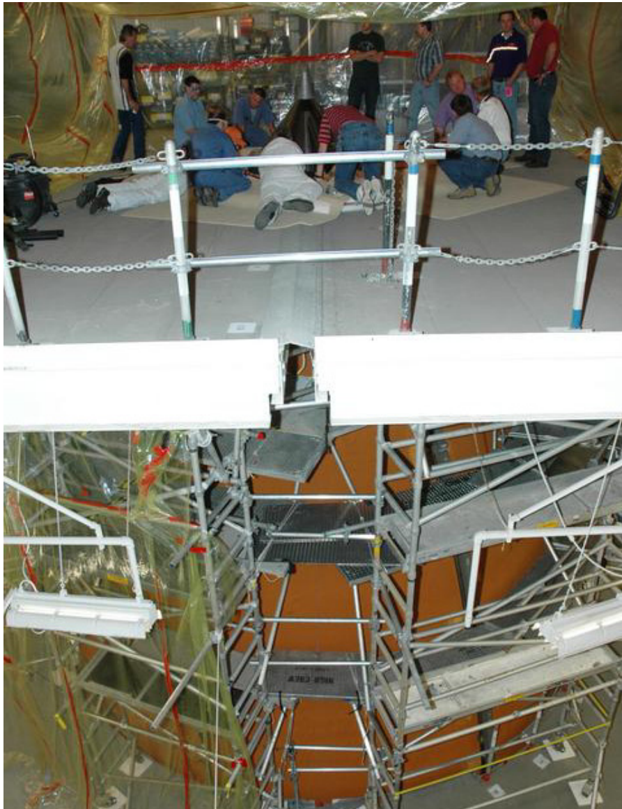
Technicians work on repair techniques to the hail-damaged external tank. They are inside a tented area that protects the tank. Scaffolding around the tank can be seen below.
